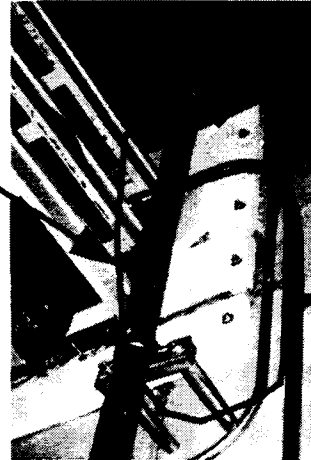
Fig.2 Wall Damage Example(2) (Calcium-silicate board PSS)
