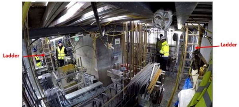
Figure 4: Cramped conditions inside the formworks.
