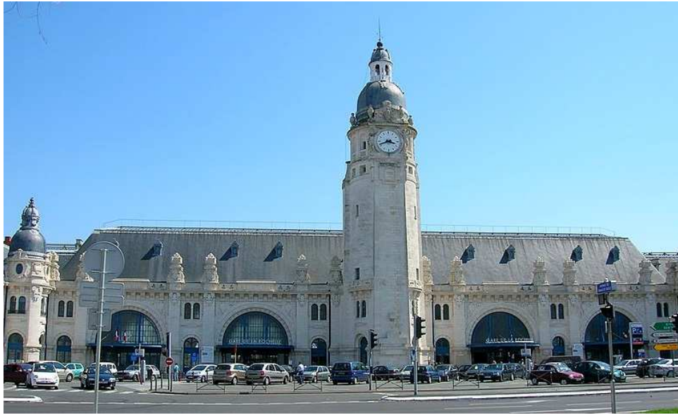
La Rochelle railway station
