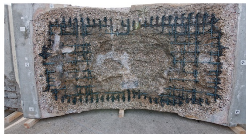
Tunnel Lining Segment after Fire Test
