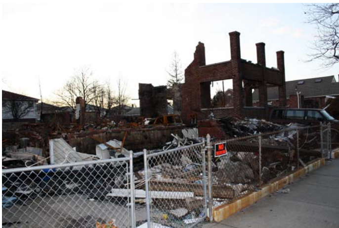
Figure 3. Photograph of Building of origin on Beach 129 Street in foreground, looking to the northwest.
