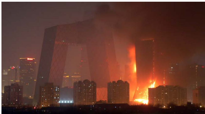
Beijing TVCC building fire during Feb. 9 2009. Photo from Wikipedia.
