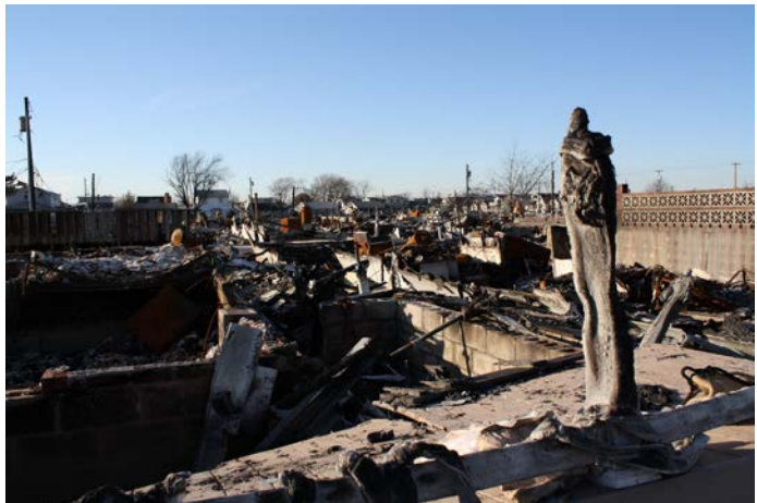
Figure 1. Damage following the fires in Breezy Point. Looking north from the area of origin.
